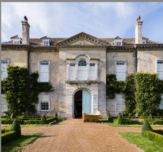
Extensive maintenance and repair programme at Firle Place
