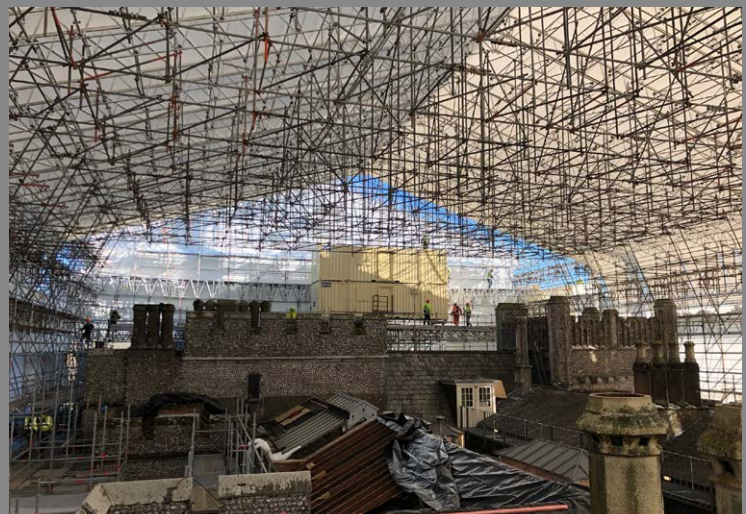
West Dean College Roof Conservation
